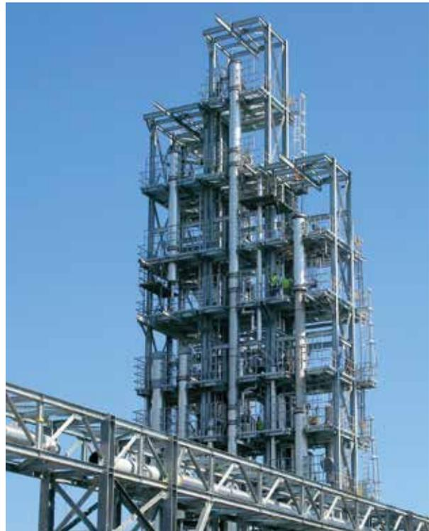
configurations. The center commissioned the PSTU and conducted several test campaigns with MEA solvent. Demonstrating mass and energy balance closures of nearly 100 percent, the testing provided a baseline regeneration energy of 1,500 to 1,720 British thermal units (BTUs) per pound (lb.) of CO<sub>2</sub>.
