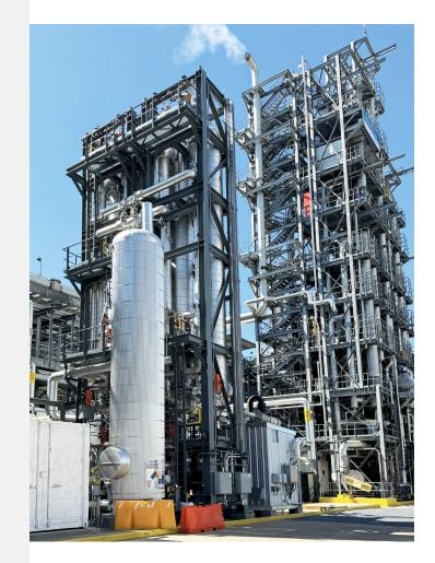
Carbon America was excited to test our new FrostCC™ technology at the National Carbon Capture Center. With an in-depth understanding of technology, the facility's highly specialized engineers and project managers enabled us to demonstrate carbon capture on natural gas flue gas successfully. Our FrostCC technology allows us to drive down capital costs of carbon capture projects to half what they are today. ■
