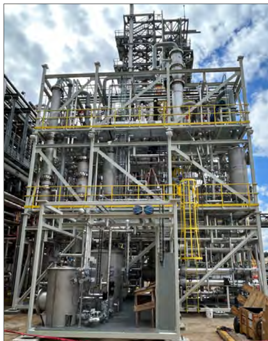
Figure 13. Installed SRI Modules
