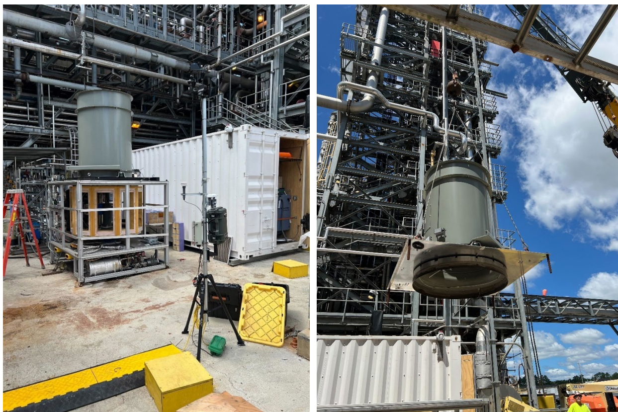
Figure 14 – DAC-100, Heat Skid, and Liquefaction container being decommissioned at the NCCC
