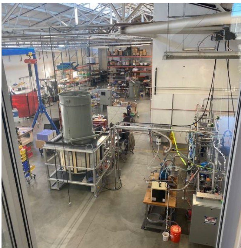
Figure 9 – Mid Construction DAC-100 and Heat Skid
