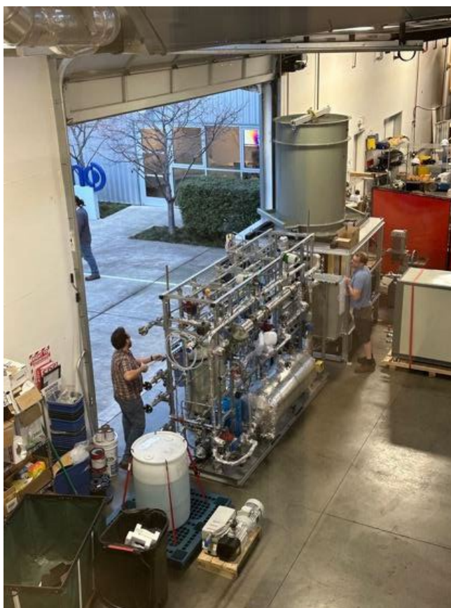
Figure 10 – DAC-100 and Heat Skid preparing for shipment from AC's Berkley facility
